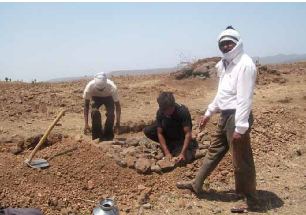
Image: Water Retention Structures
