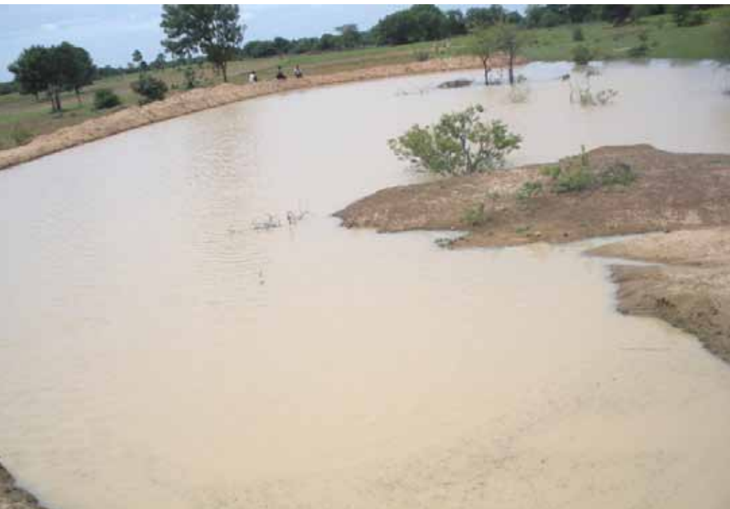
Image: Rain Water Storage Pond
